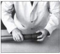
**Note:** For pipe sizes 6" and larger, two people will be required, a mechanical forcing device should be used, and the joint should be held together for up to 3 minutes.
