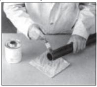
Apply a medium layer of cement to the fitting socket. Do not let the cement puddle. Also, when joining belled-end pipe,
