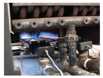
Parker's Premix Metal Fiber Burner System Shown burning and achieving better than 12ppm NOx. Standard units achieve 20-30ppm NOx as required by SCAQMD.
